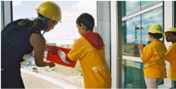
Young Consultants at the launch of Architecture Week 2004 at the Unicorn Theatre construction site. Courtesy: Bonnie Smith
